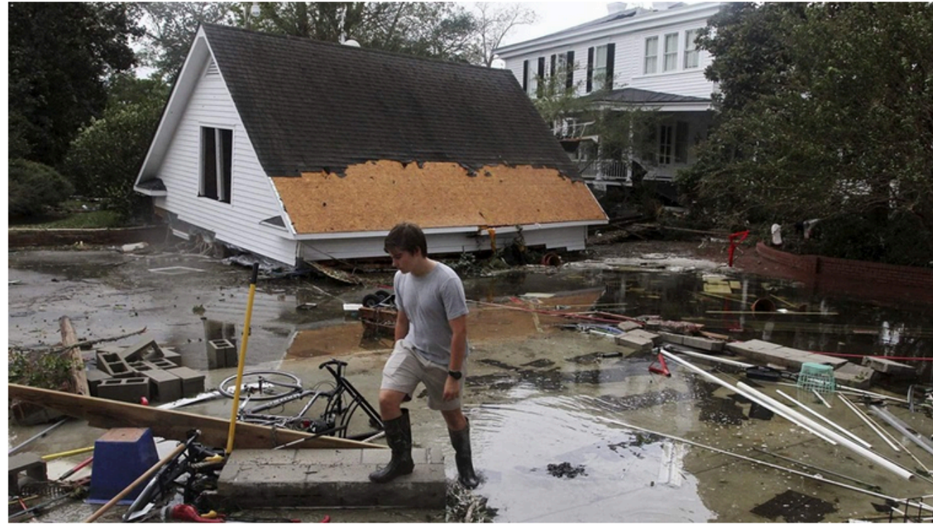
Resident Joseph Fudi looks at flood debris and storm damage from Hurricane Florence at a home in New Bern
